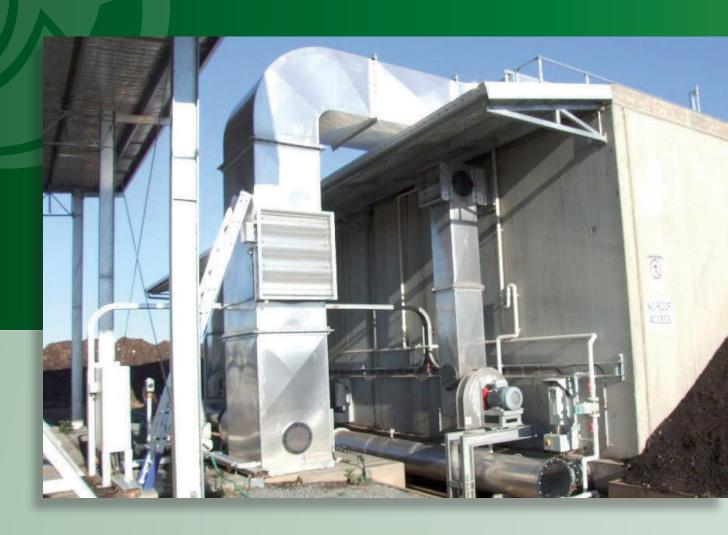
We have three tunnel bio-reactors at our Shepparton facility, each with a capacity of 350-400 cubic metres. The 25m-long concrete tunnels are serviced by a forced air system to maintain the oxygen level throughout the process. A process water system maintains correct moisture levels for efficient microbial activity.
