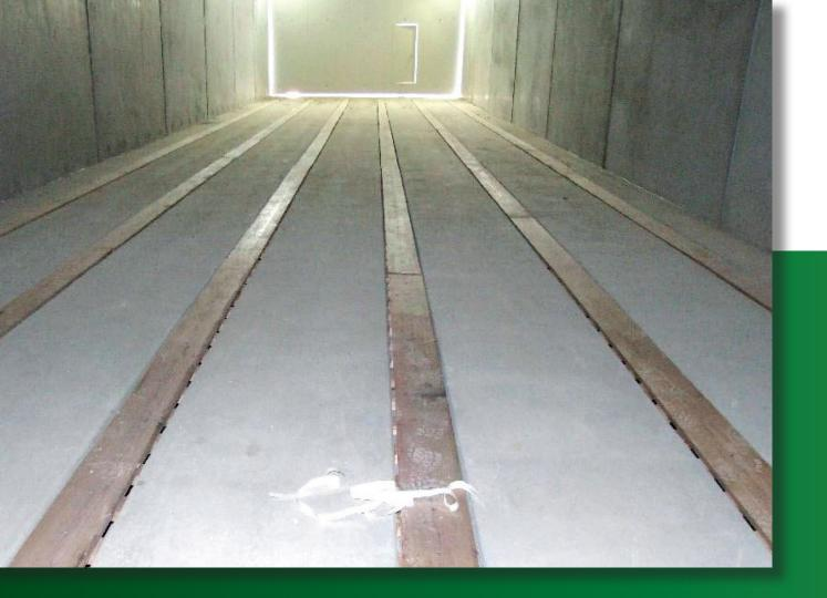
Each day, we load sorted green waste feedstock into the vented tunnels using a front-wheel loader. To prevent odour escape we keep the tunnels under negative pressure.
